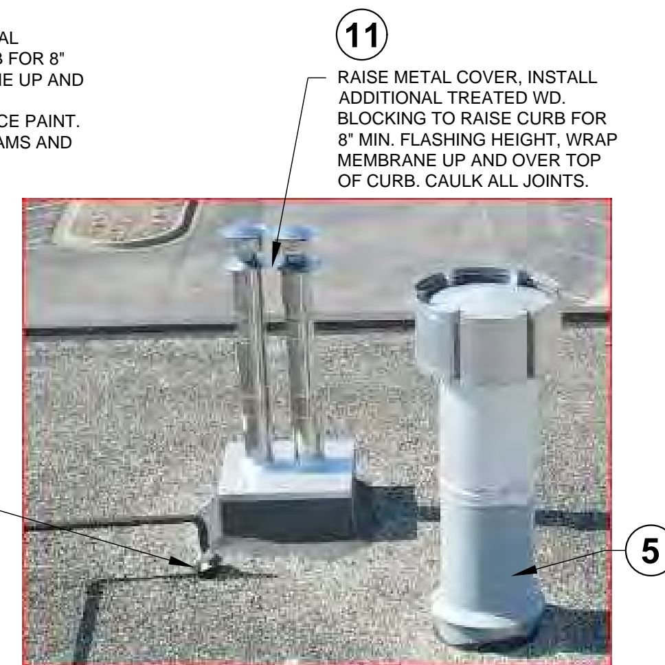
11 FLUE CHASE DETAIL SCALE: NTS
