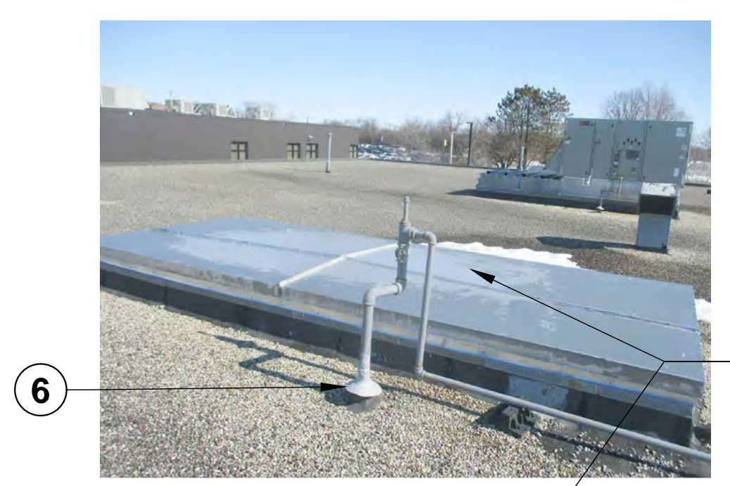
6 PITCH PAN DETAIL SCALE: 1-1/2" = 1'-0"
