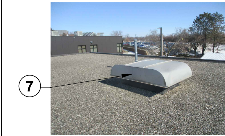
8 EXISTING CURB MOUNTED UNIT TO REMAIN. CUT EXISTING FLASHING; SEAL CORNERS, LAP OVER NEW FLASHING. EXISTING SHEET METAL COVER TO REMAIN. NEW SHT. MTL. SLIP FLASHING WITH MECHANICAL FASTENERS AND GASKETED WASHERS @ 12" O.C. NEW BUTYL TAPE AT TRANSITION. NEW CANT STRIP. NEW FULLY ADHERED FLASHING MEMBRANE TUCKED BEHIND EXISTING FLASHING. NEW ROOFING AND INSULATION ASSEMBLY. EXISTING ROOF DECK.
