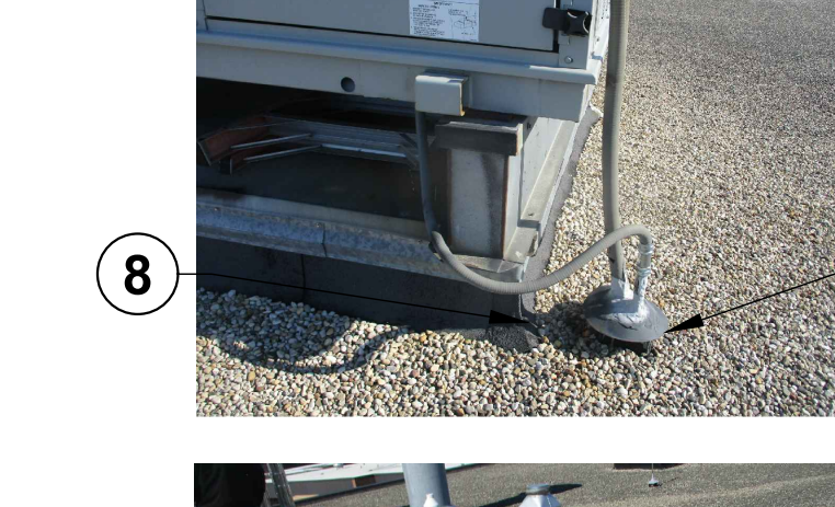
8 EXISTING CURB MOUNTED UNIT TO REMAIN. CUT EXISTING FLASHING; SEAL CORNERS, LAP OVER NEW FLASHING. EXISTING SHEET METAL COVER TO REMAIN. NEW SHT. MTL. SLIP FLASHING WITH MECHANICAL FASTENERS AND GASKETED WASHERS @ 12" O.C. NEW BUTYL TAPE AT TRANSITION. NEW CANT STRIP. NEW FULLY ADHERED FLASHING MEMBRANE TUCKED BEHIND EXISTING FLASHING. NEW ROOFING AND INSULATION ASSEMBLY. EXISTING ROOF DECK.
