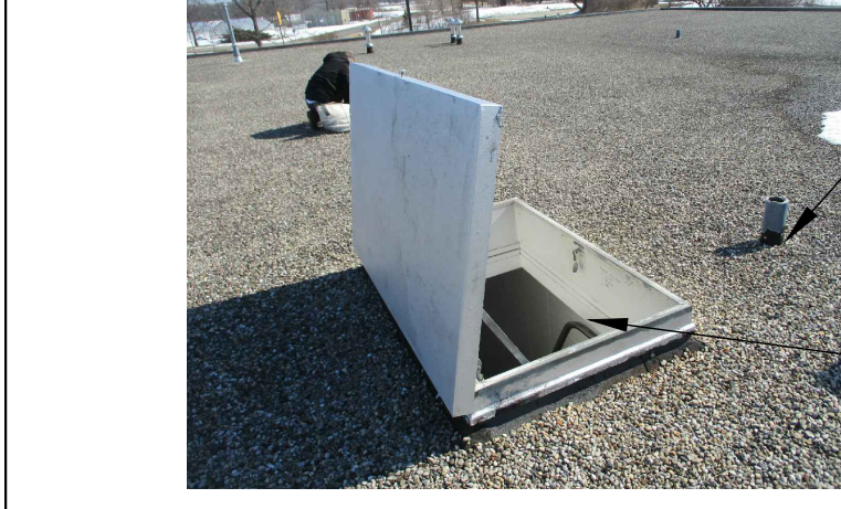
8 ABANDONED PENETRATION: REMOVE EXISTING COVERICAP, INSTALL PLATE OVER DECK OPENING.
