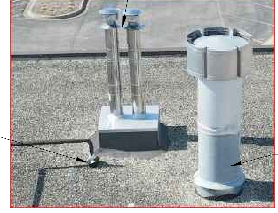
5 RAISE METAL COVER, INSTALL ADDITIONAL TREATED WD. BLOCKING TO RAISE CURB FOR 8" MIN. FLASHING HEIGHT, WRAP MEMBRANE UP AND OVER TOP OF CURB. CAULK ALL JOINTS.
