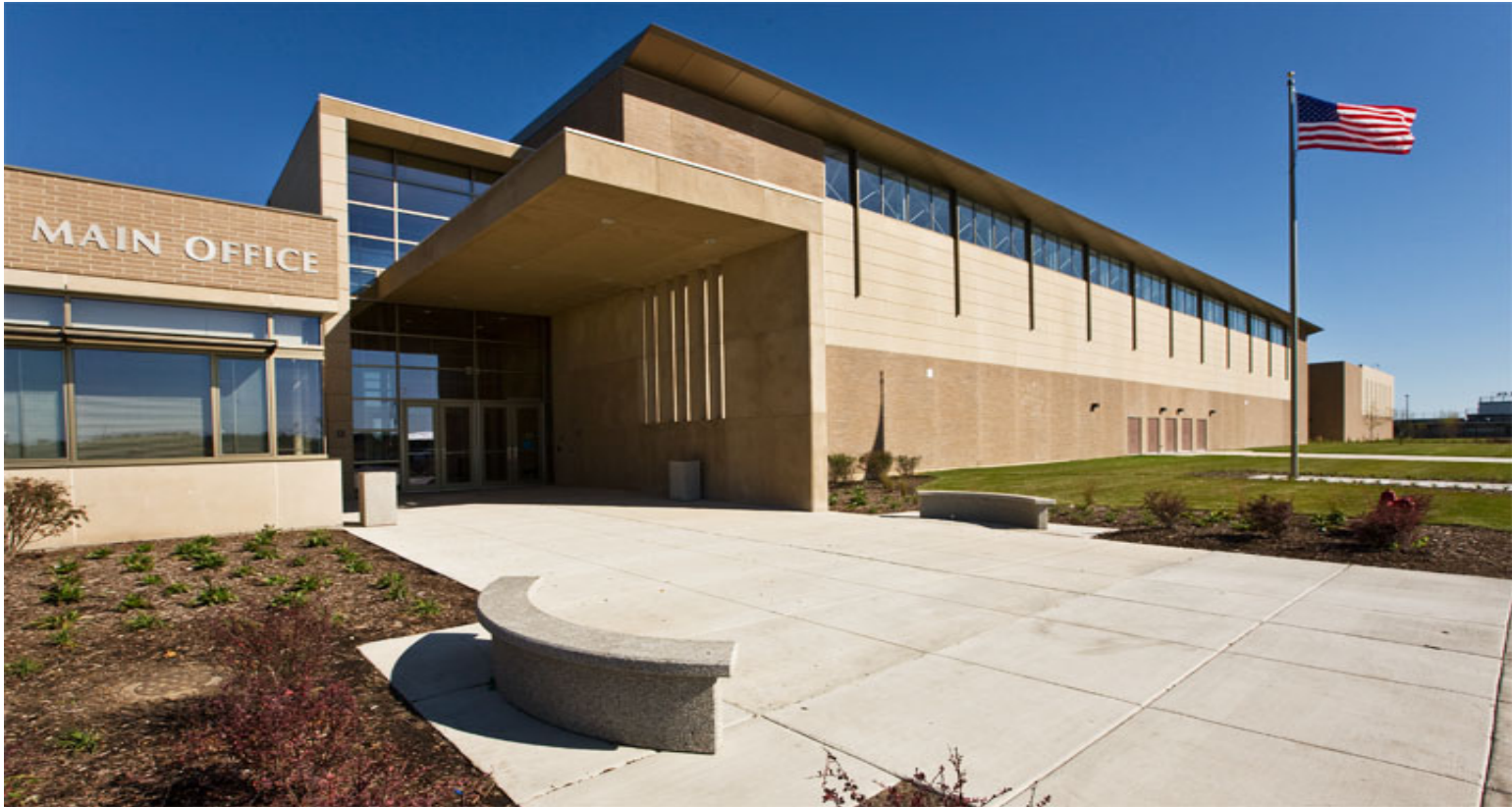
Woodstock North High School 3000 Raffle Road, Woodstock, Illinois Owner: Woodstock Community Unit School District 200 Date: 10-09-08 View: File: 18473-333prt Photo By: McShane-Fleming Studios, Chicago
